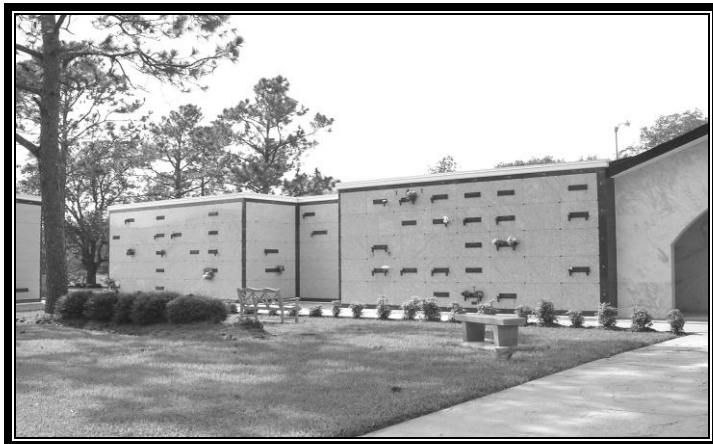
The south wing of the mausoleum.
